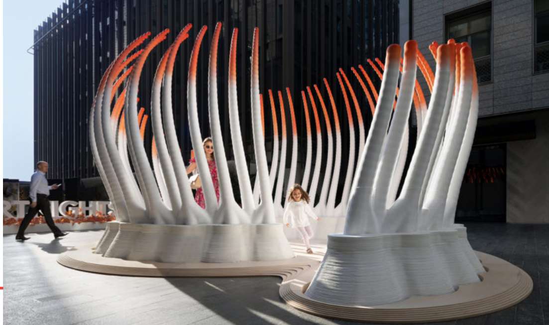
Legend: 3D Printed pavilion made from recycled plastic bottles – Credit NAARO
